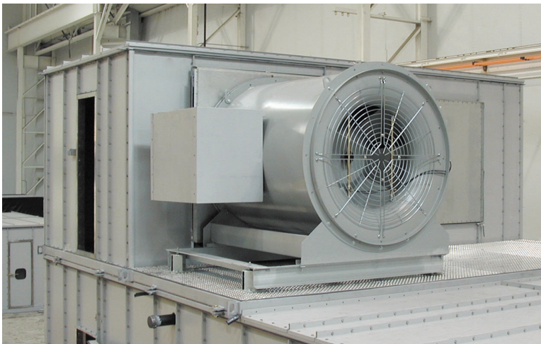
A mixed flow fan was mounted on the second tier of each primary unit, making it possible to duct return air directly to the fan (above).
